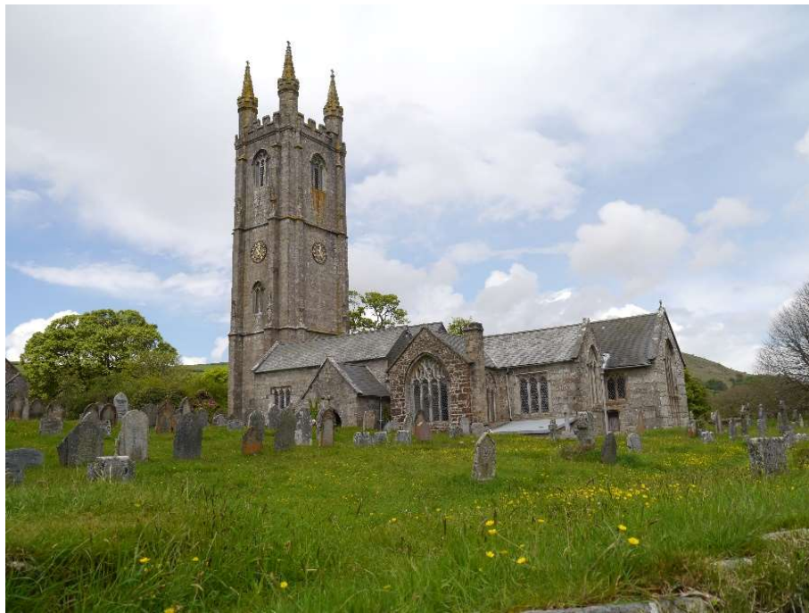
Abbildung 13 - St. Pancras Church, Widecombe in the Moor (14. Jhdrt) xiii
